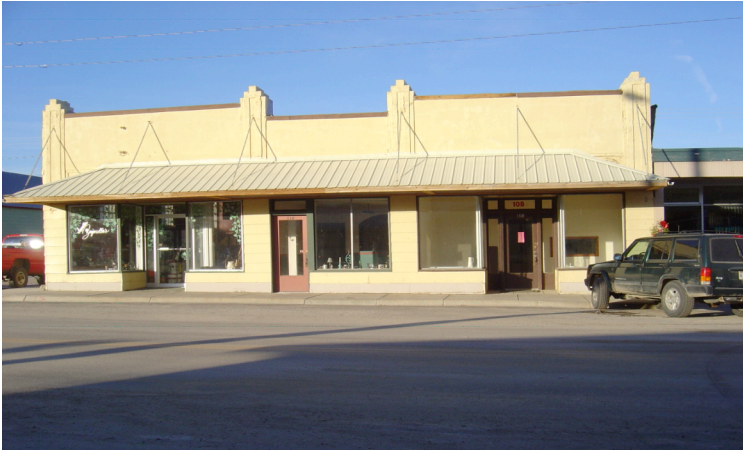
Figure 4: One Story Stucco Building in Central Business District
